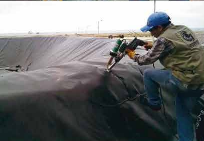
▲ Repairing Geomembrane LST610B
