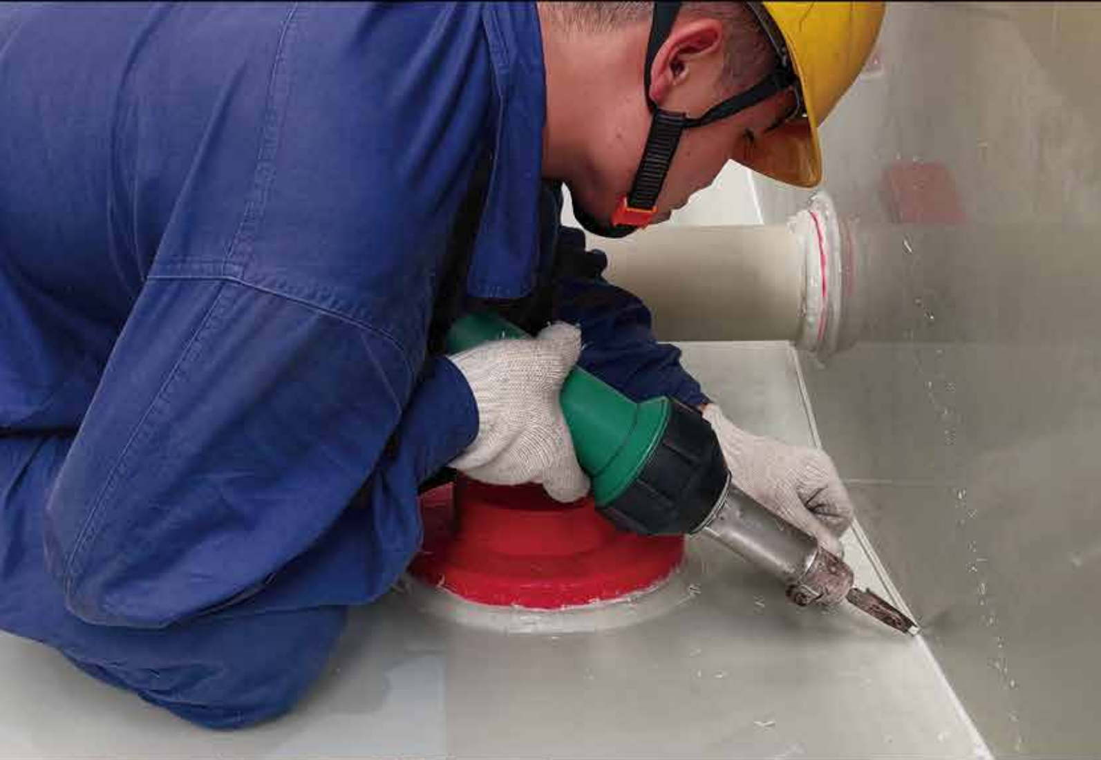
▲ Welding PP plate for inner Lining of Carriage LST1600S
