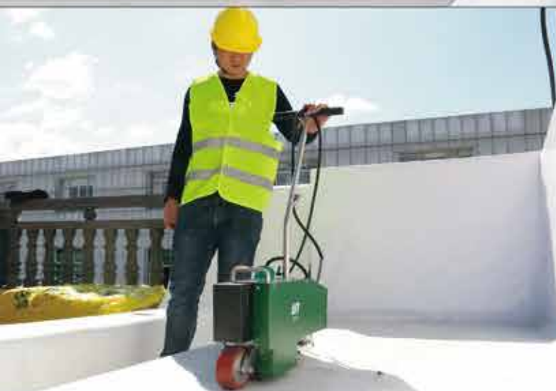
▲ Fast and efficient welding of TPO LST-WP1
