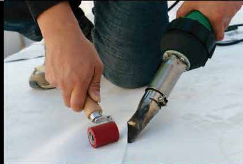
▼ Welding TPO Membrane in Roof, LST1600S
