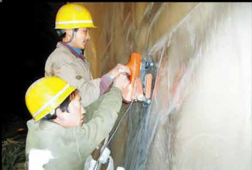
▼ Tunnel Waterproofing Sheet Welding LST800
