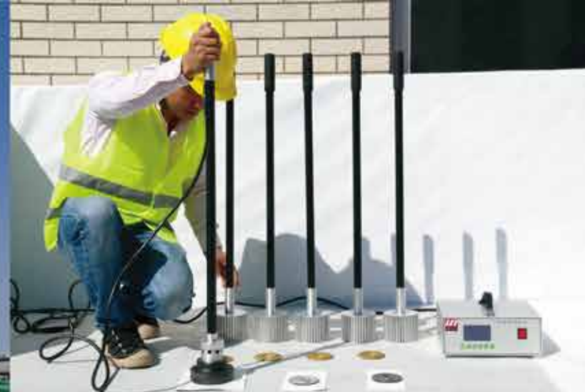
▲ Non-perforation welding of membrane and fastening gasket realized by magnetic welding machine LST-REW
