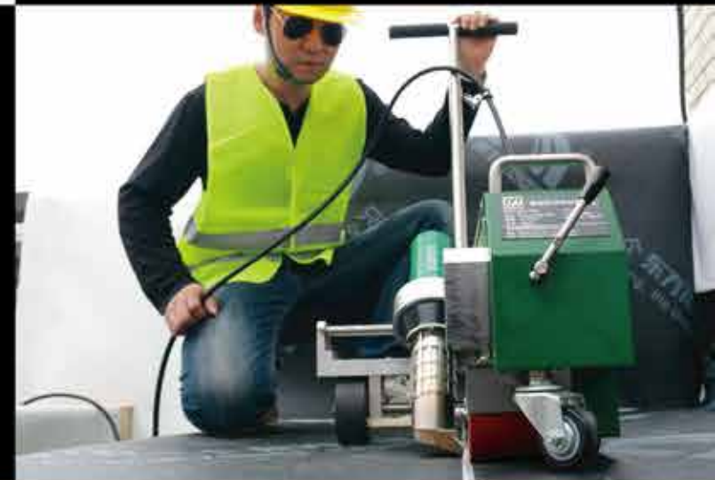
▼ Welding modified SBS by flameless method LST-WP2
