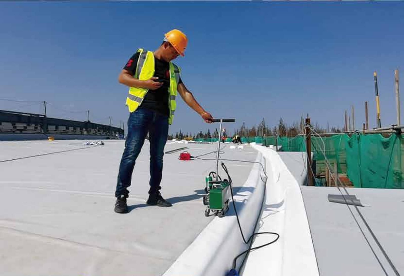
▲ Gutter edge welding LST-WP4
