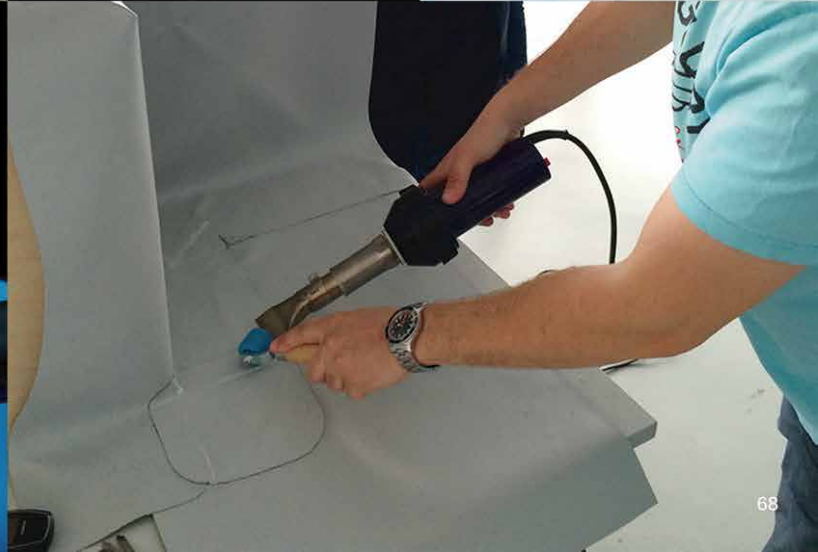
▼ Repairing and Welding the Internal and External Angles of Roof TPO Membrane LST1600A
