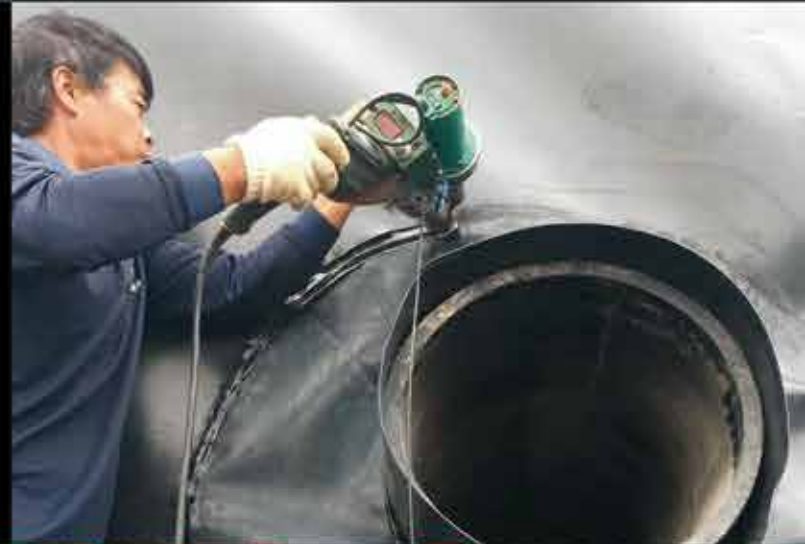
▼ Welding HDPE membrane to Pipe LST610A
