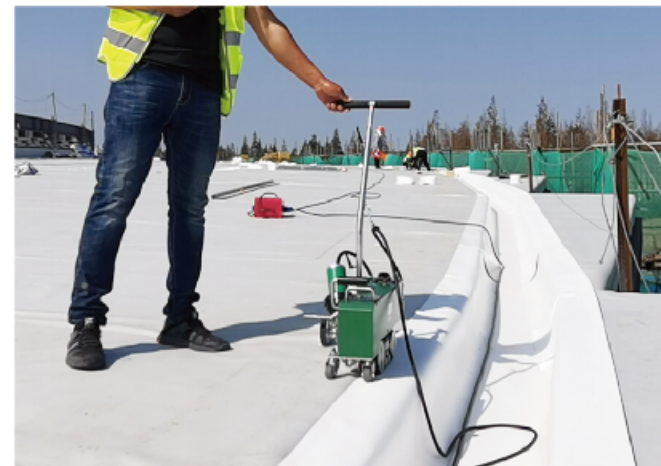
Gutter Edge Welding LST-WP4
