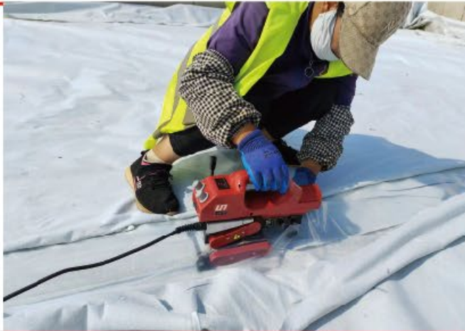
Composite Material Solid Waste Landfills LST800D
