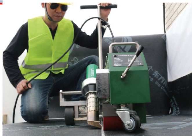
Welding Modified SBS by Flameless Method LST-WP2
