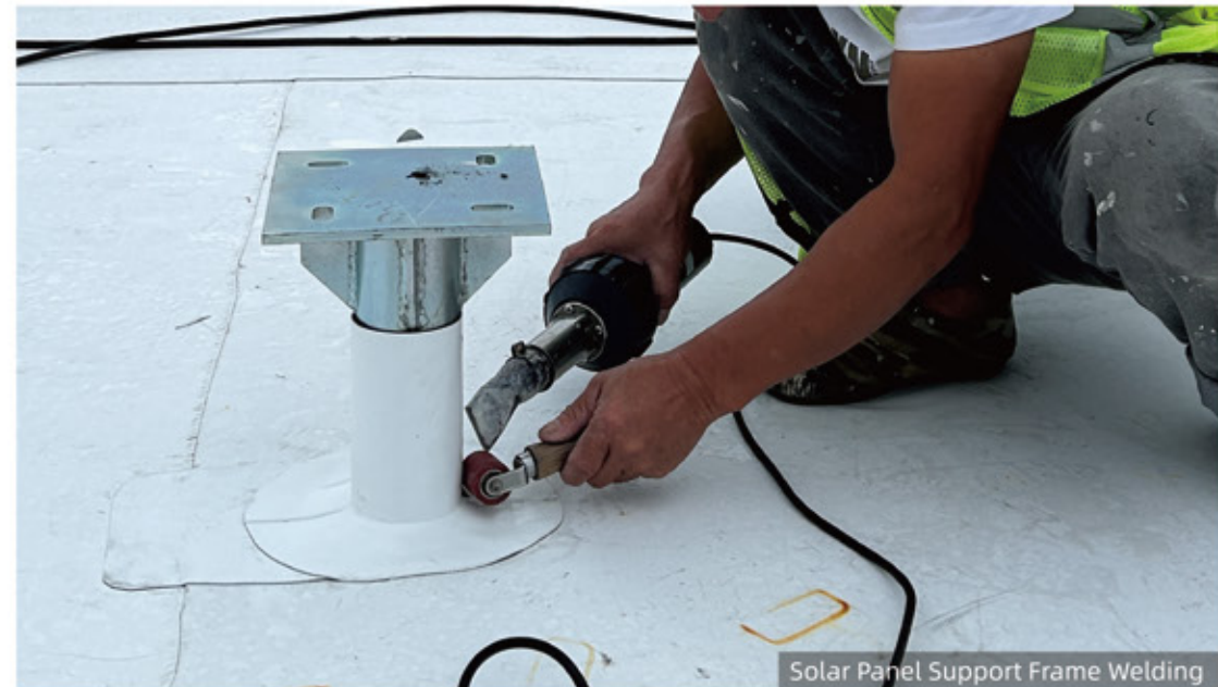
Photovoltaic Bracket Welding
