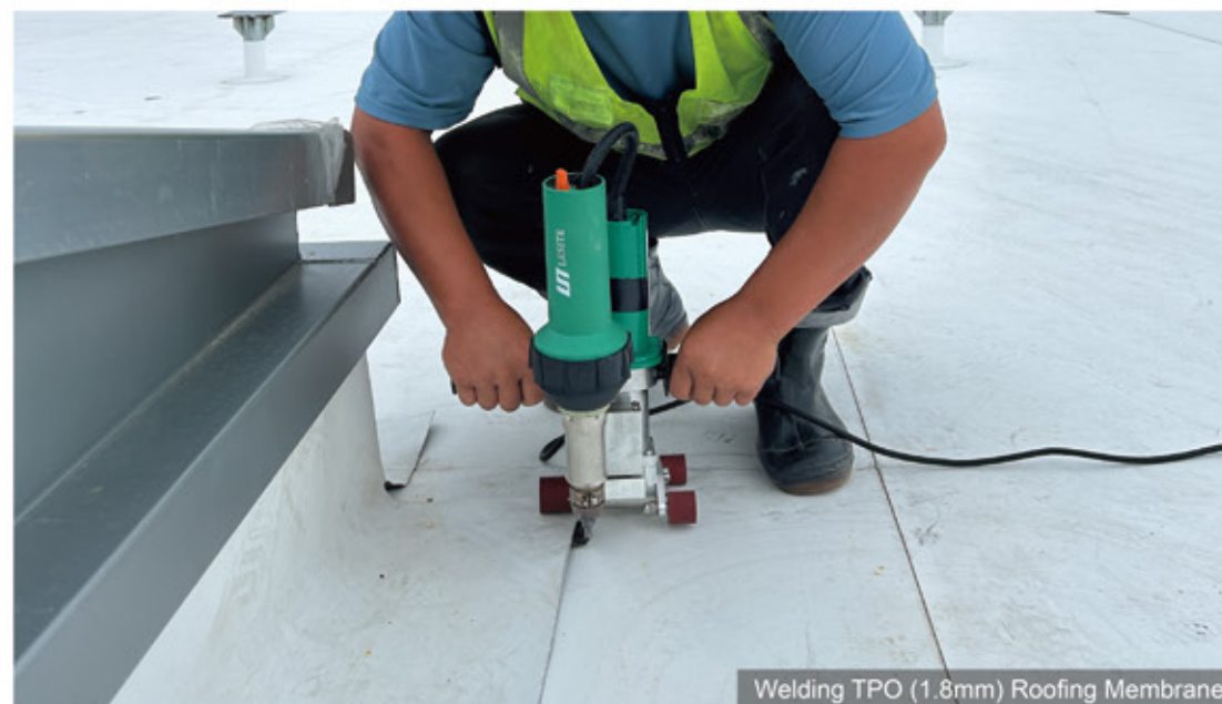
Welding TPO (1.8mm) Roofing Membrane
