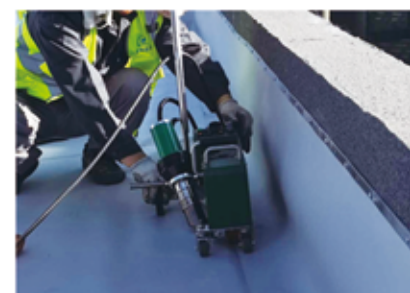
Parapet Wall Welding
