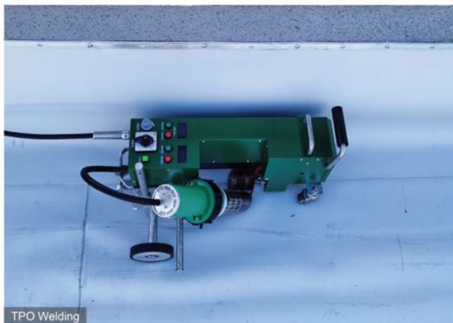
Fast and Efficient TPO Welding
